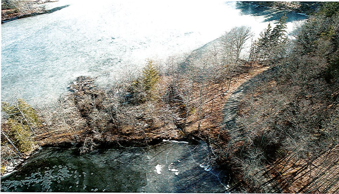
Middle South Lake dam looking south.
