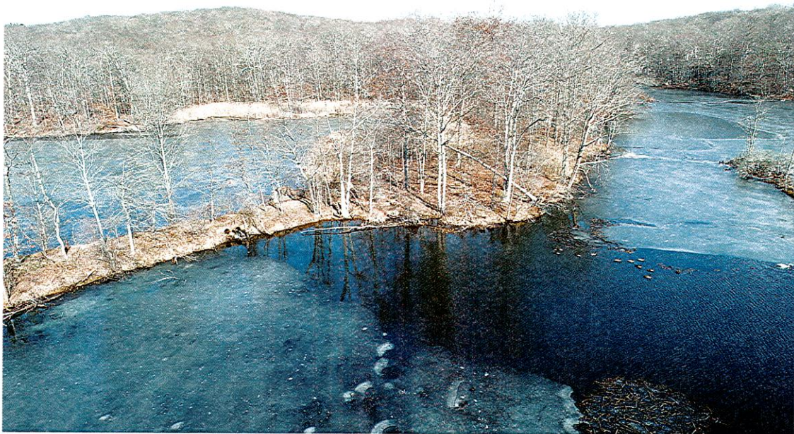
Upper South Lake dam looking north.
