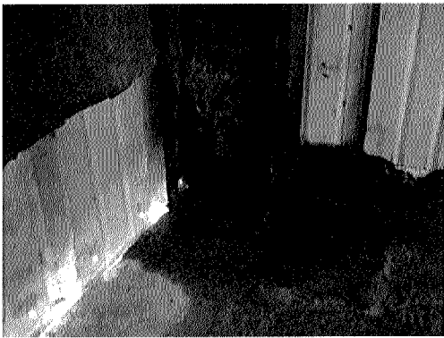
Failing Gable Column and Base Angle
