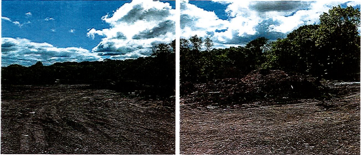
Old separation operation area being cleared (refer to 1/31/18 and 4/16/19 Site Visit Reports for photos of previous operation.) Piles of sand; wood chips; mixed asphalt, concrete, rock, and soil; and large rocks have been removed.
