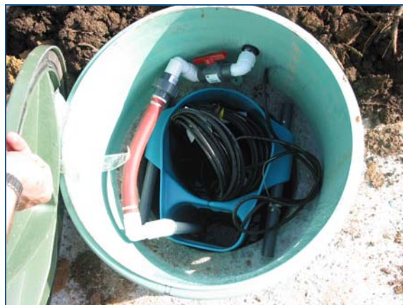
In a STEP system, an effluent pump is installed within a pump vault in the outlet end of a septic tank.
